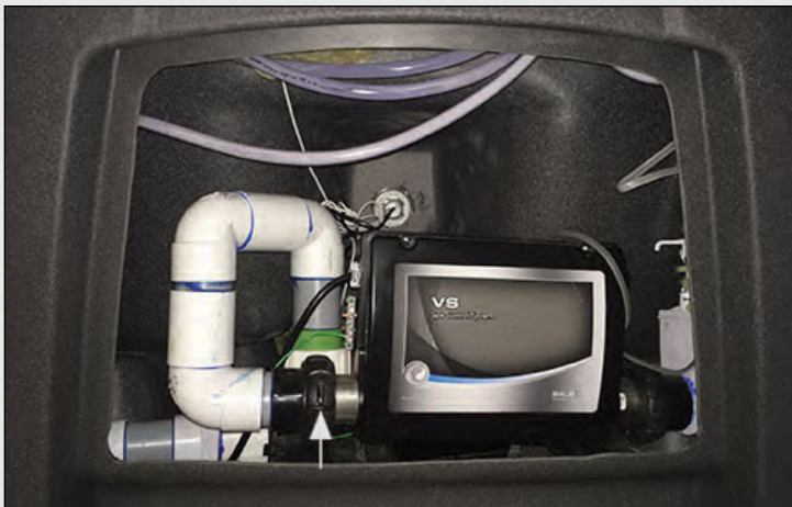
FIGURE 1.2a : HEATER UNION; LOOSEN UP TO BLEED AIR
